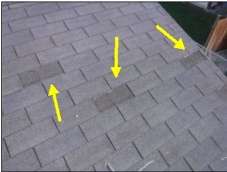
missing shingles
