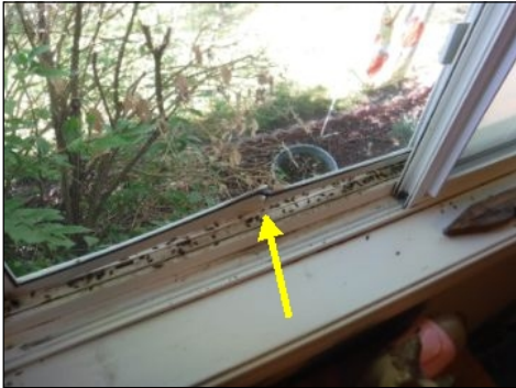
screen frame damaged
