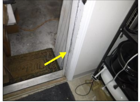
weather stripping cracked or damaged
