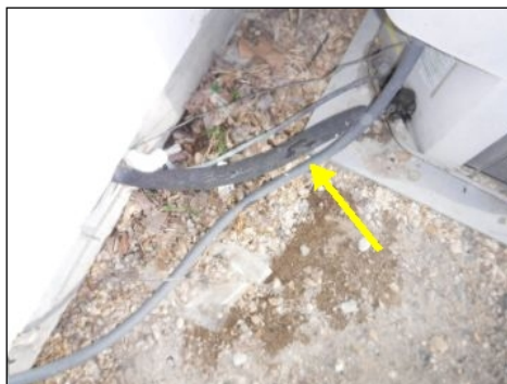
damaged insulation
