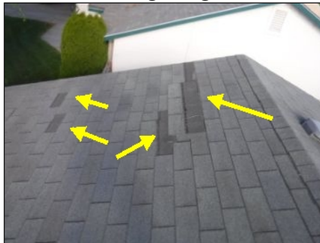
missing shingles
