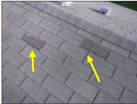
missing shingles
