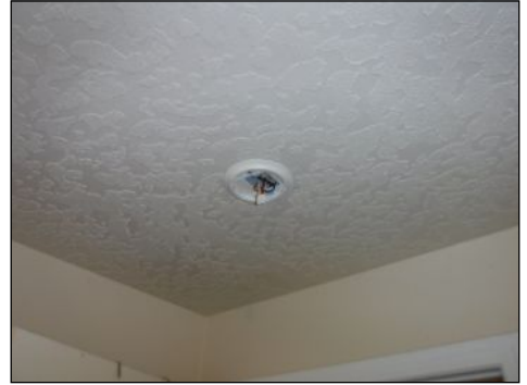
missing smoke detector
