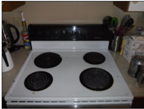
no anti-tip bracket installed
