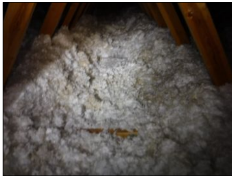
insulation compressed or disturbed
