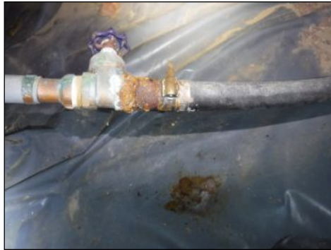
corroded fitting and past leaking
