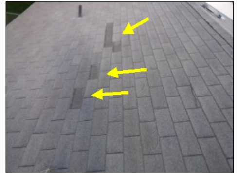
missing shingles
