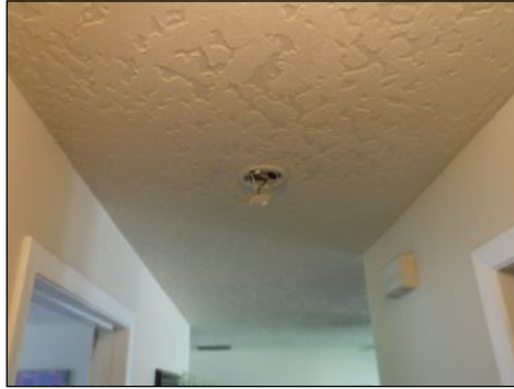
missing smoke detector
