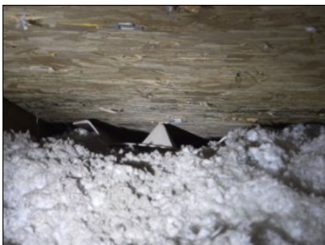
attic baffles are properly installed
