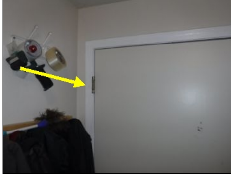
self closing hinge on garage door needs adjustment
